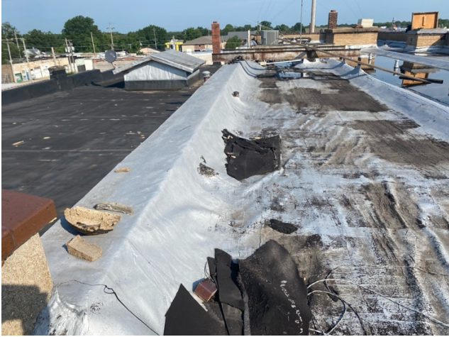
Roof looking South
