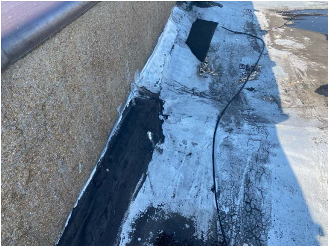
Close up of parapet wall
