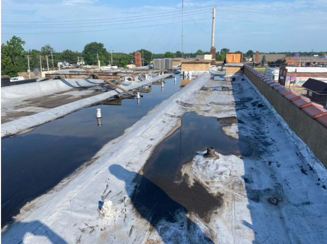
Roof looking North
